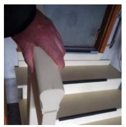
Remodeler Dave Matthews mounted an easy-tograsp grip rail on top of the 2x6 handrails, added sand to the tread paint to improve traction, and applied contrasting nonslip tape to the nosings to help with visibility.
