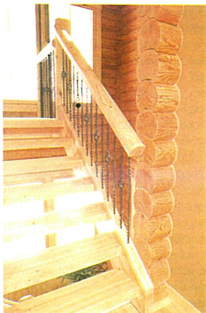
ABOVE & BELOW: The stairway is a focal point. It has tall windows facing the trees. As you go upstairs, you have a nice vista. It’s built of log and seems to speak to the solidity of the materials. The stair is suspended on steel tubing. Rods go through the treads to allow for settling. The stairs not only function well but turned out to be an eye-catching design element of the home.
