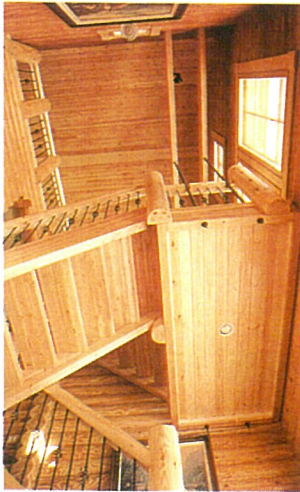
ABOVE & BELOW: The stairway is a focal point. It has tall windows facing the trees. As you go upstairs, you have a nice vista. It’s built of log and seems to speak to the solidity of the materials. The stair is suspended on steel tubing. Rods go through the treads to allow for settling. The stairs not only function well but turned out to be an eye-catching design element of the home.
